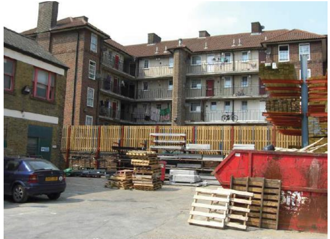
2 LOOKING NORTH FROM WITHIN THE SITE TOWARDS HOLLYBUSH HOUSE
